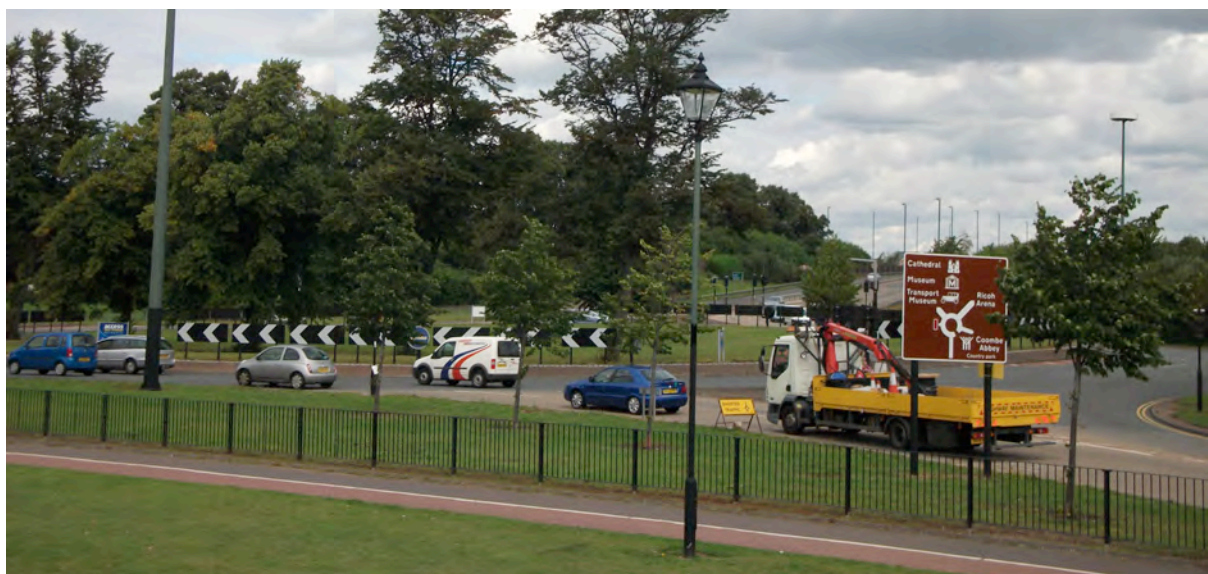
Figure 2; Junction of the A444/Binley Rd, Coventry.
